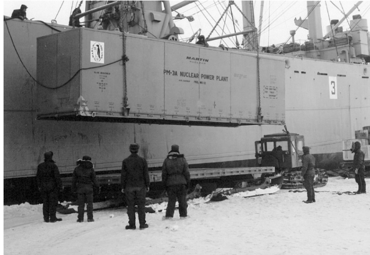
Figure 1 PM-3A reactor components arriving by ship at McMurdo Station, Antarctica
